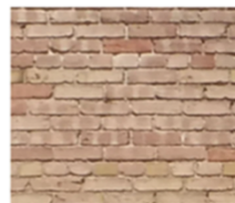
EXISTING BRICK NATURAL
