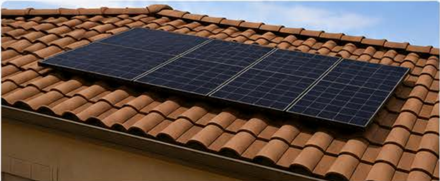
Mounted parallel to roof slope.
