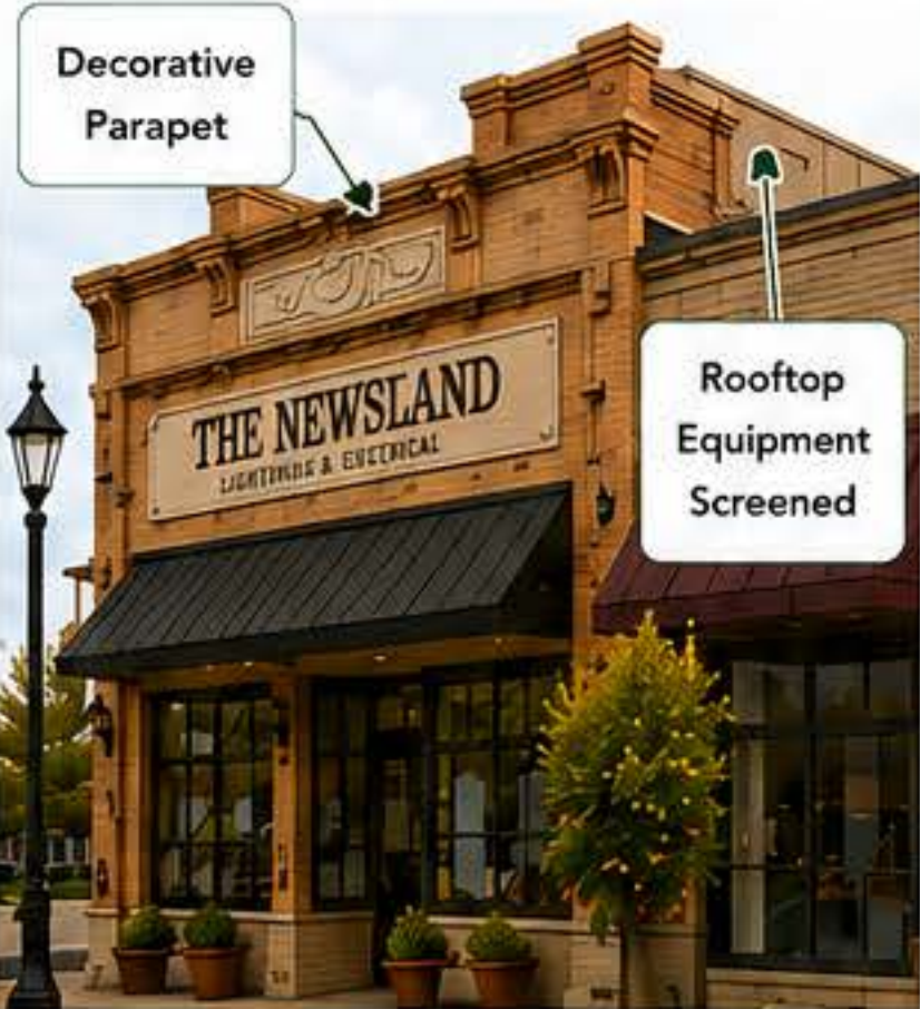
Parapets and cornice treatments add definition and screen rooftop equipment.
