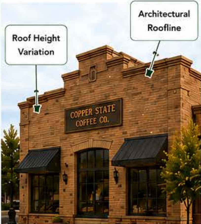
Variations in roof height create visual interest and reduce building mass.
