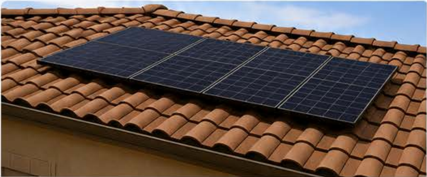
Mounted parallel to roof slope.
