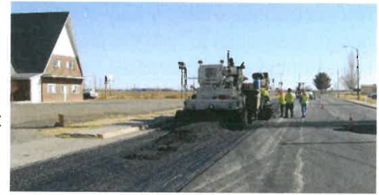
Construction Administration: Our team handles construction administration for the City of Winslow, such as this Route 66 Pavement Maintenance project.
