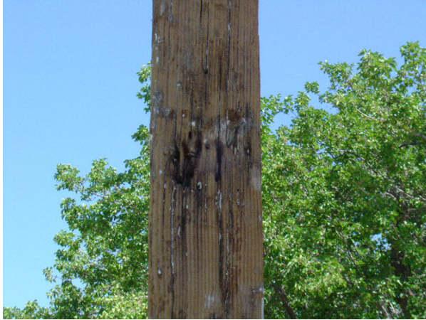
Termite damage
