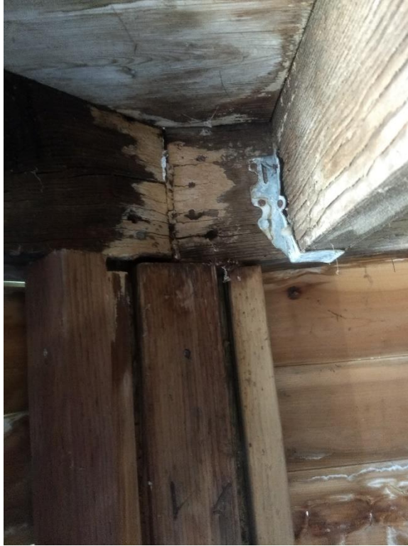
Figure 5: Rim joists at corner post.
