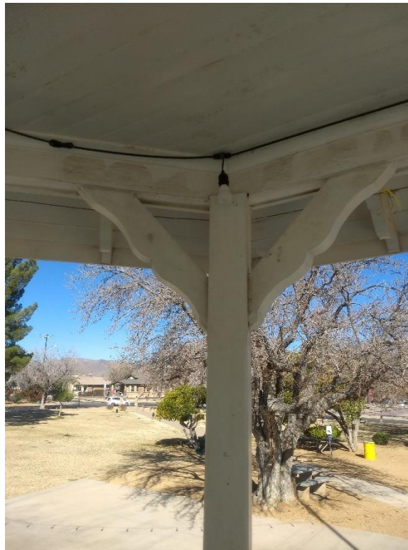
Figure 2: Beam, knee brace, and post connection.
