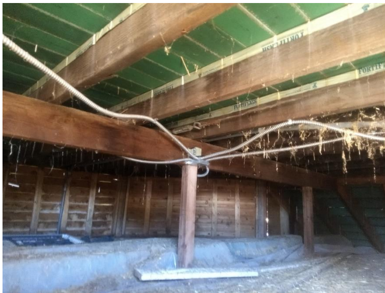
Figure 4: Floor framing.
