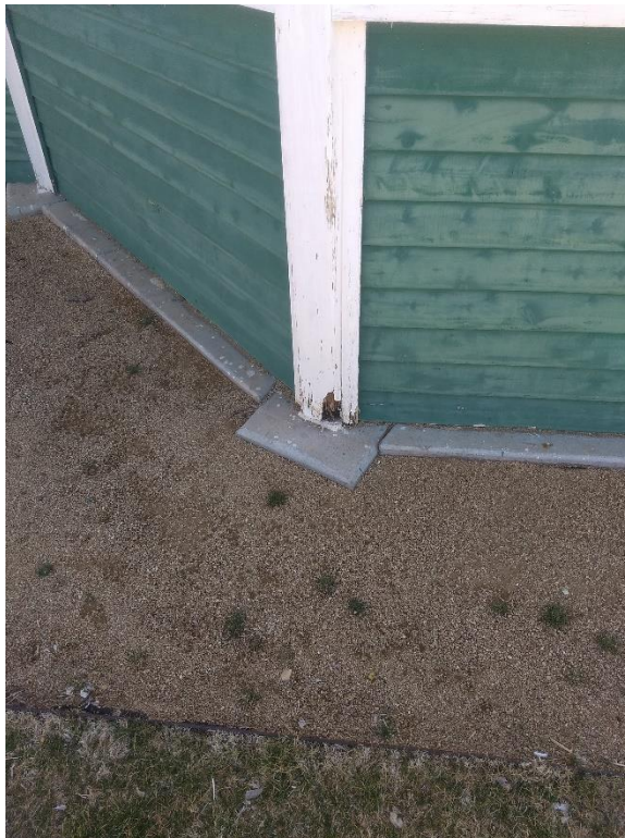
Figure 6: 6x6 wood post at foundation.
