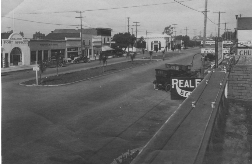
Figure 1. 1926 view of the Third Avenue district.
