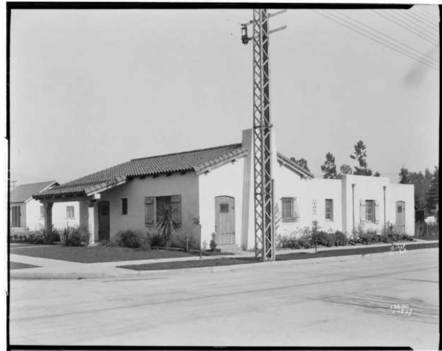
Figure 8. SCE Ramona Substation, built in 1926 in a Spanish Revival style to blend into the surrounding residential tract.
