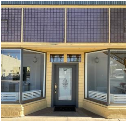
Example of Clerestory Windows & Transom Windows on Main Street
