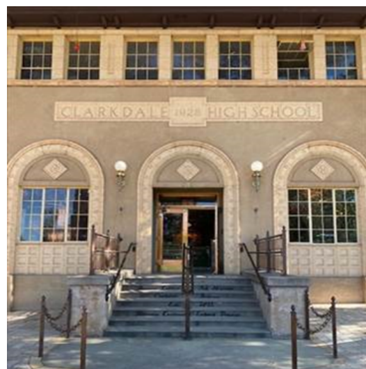
Example of an Arched Entry
