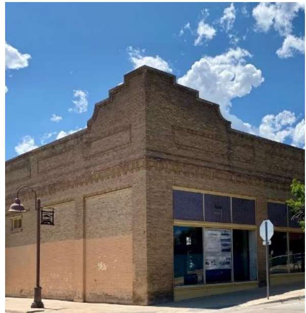
Example of Parapet Wall on Main Street
