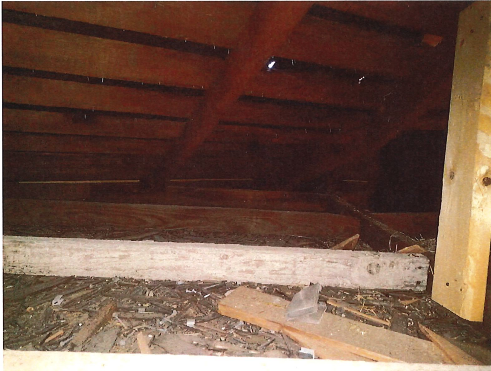
Photo 3 – Ceiling rafters and roof structure
