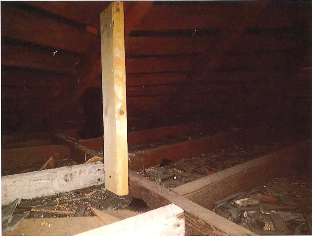
Photo 4 – post in ceiling
