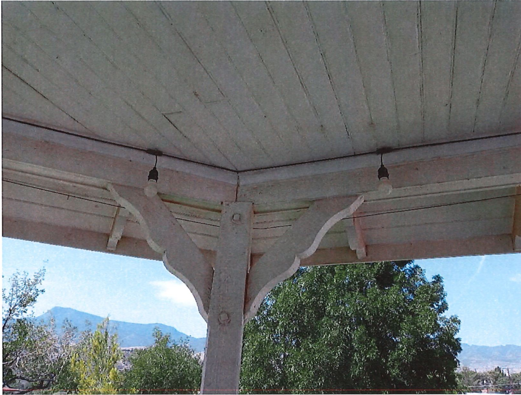
Photo 7 – View of Ceiling Lath and Column with knee bracing
