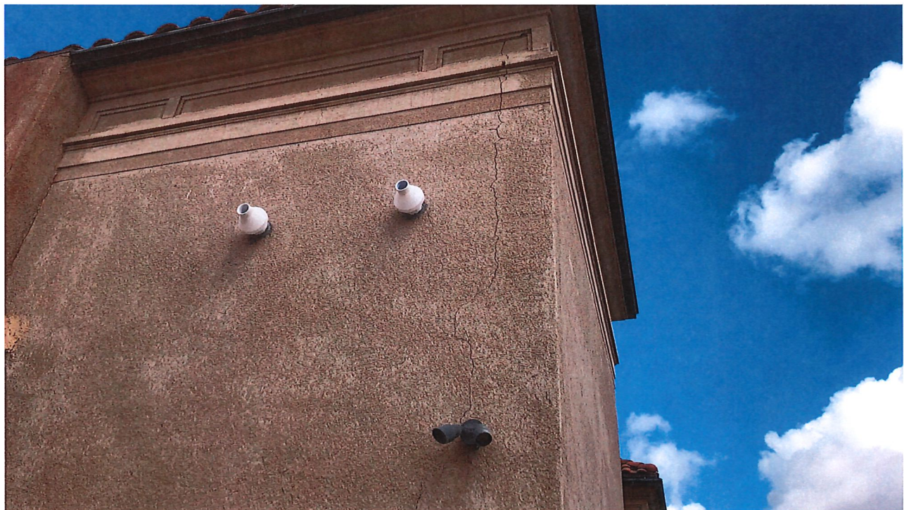
Photo 6 – Crack at Corner of Memorial Building (East Side)
