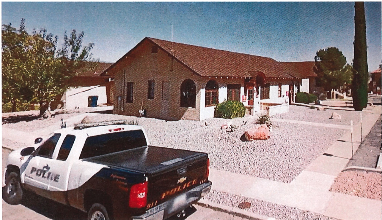
Photo 17 – Police Dept. Building
