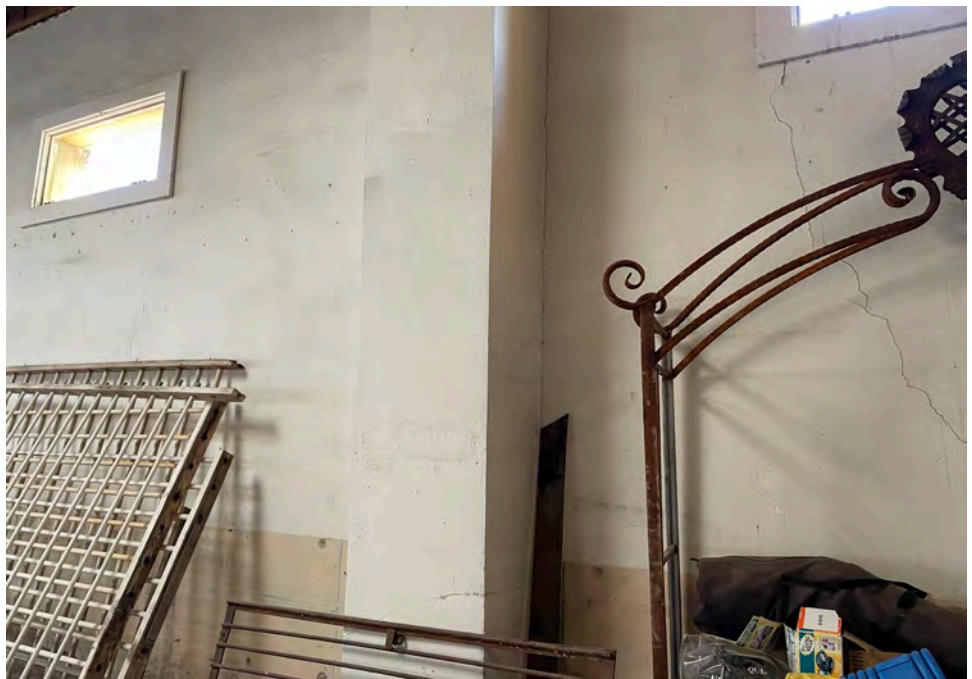
Photograph 4: Photo of LBP of B wall and window frames.
