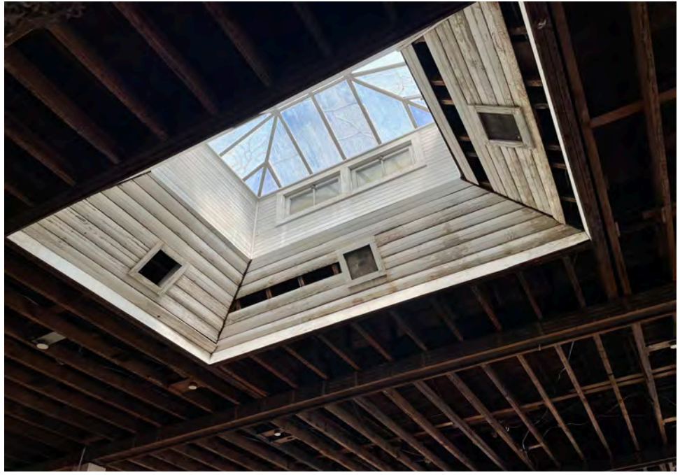
Photograph 7: Photo of LBP skylight.
