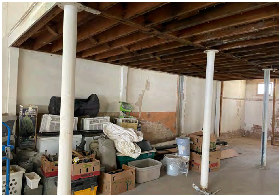
Photograph 6: Photo of LBP metal support pillars.
