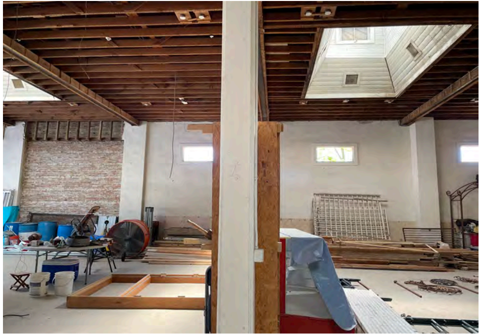
Photograph 5: Photo of LBP wood pillars.
