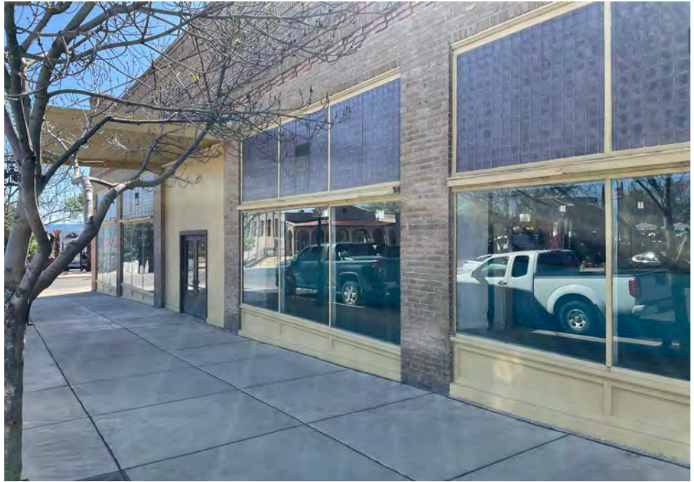
Photograph 1: Photo of LBP window trim, double doors, and window ledges.
