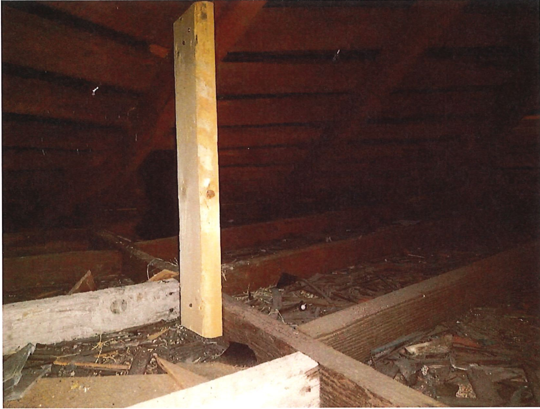
Photo 4 – post in ceiling
