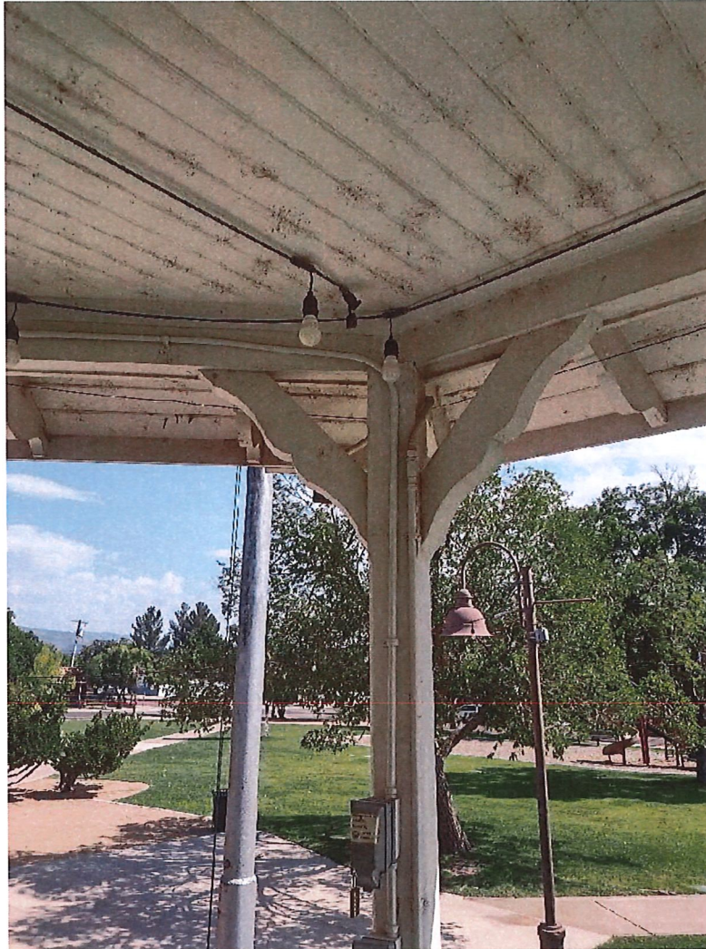
Photo 6 – View of Ceiling Lath and Column with knee bracing
