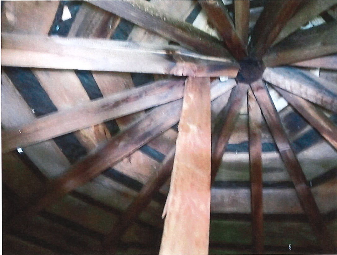
Photo 2 – Center of Underside of Roof
