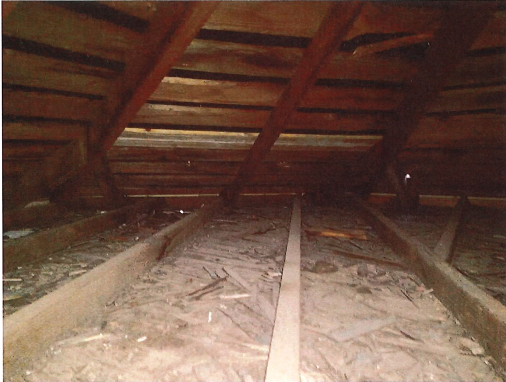
Photo 5 – Ceiling rafters and roof structure
