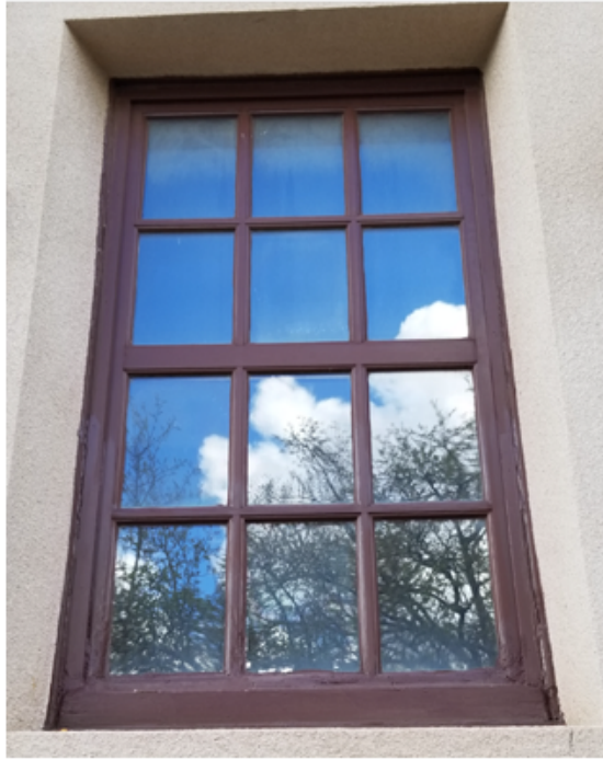
Figure 7 Replacement window- CDD Building North side
