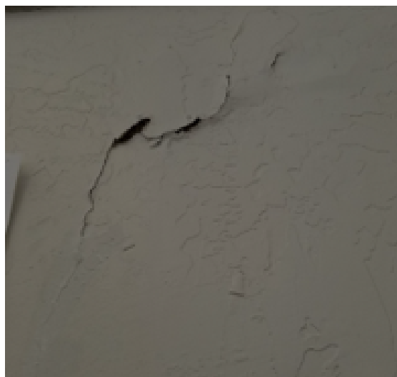
Figure 3 Plaster damage
