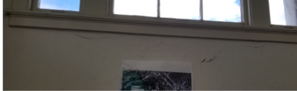
Figure 5 Public Works Supervisor's Office
