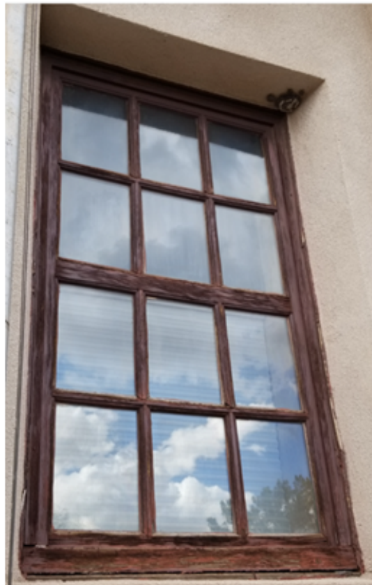
Figure 8 South side CDD building – replacement window
