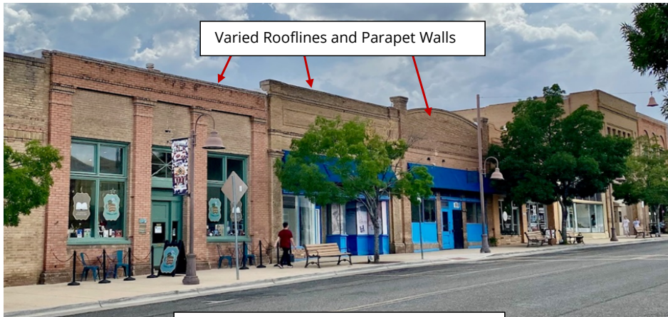
Exhibit 4: Rooflines and Parapet Walls
