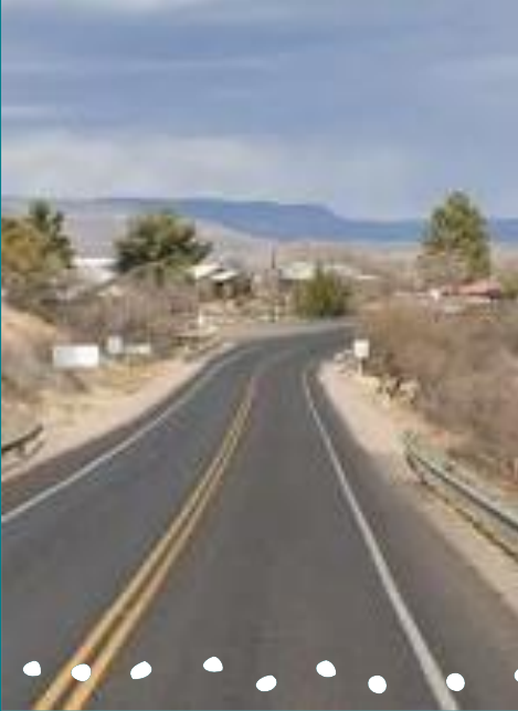
Clarkdale Parkway Sidewalks & Bike Lanes
