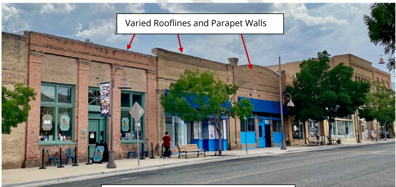
Exhibit 4: Rooflines and Parapet Walls
