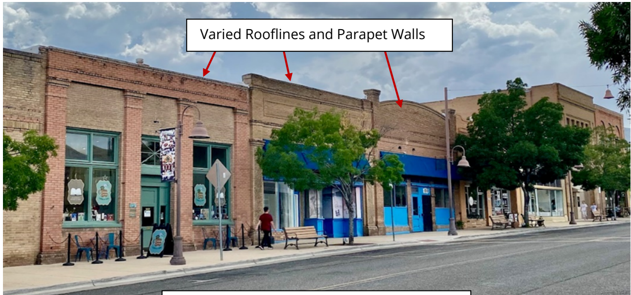
Exhibit 4: Rooflines and Parapet Walls
