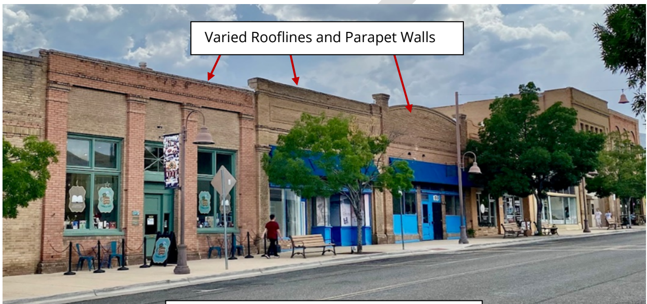
Exhibit 4: Rooflines and Parapet Walls
