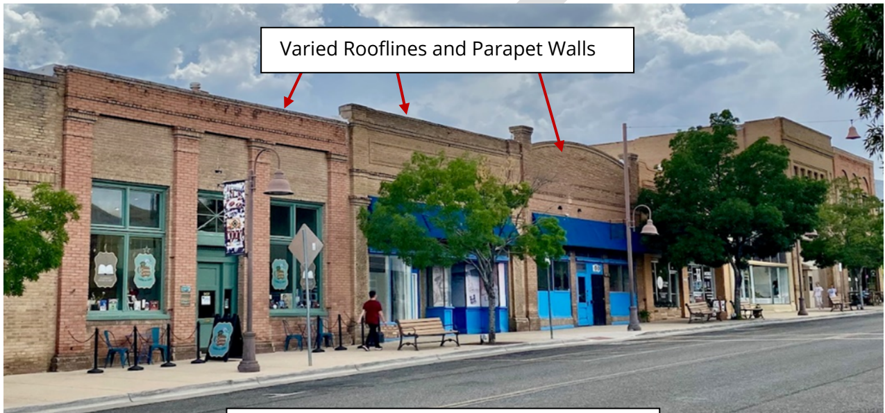
Exhibit 4: Rooflines and Parapet Walls
