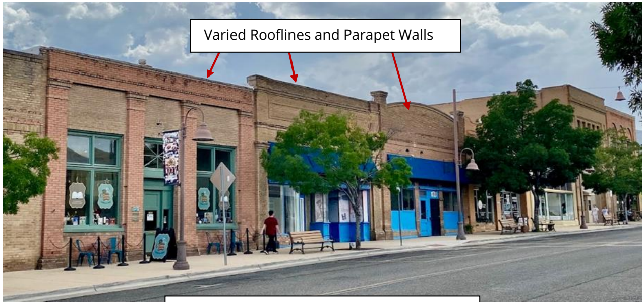
Exhibit 4: Rooflines and Parapet Walls
