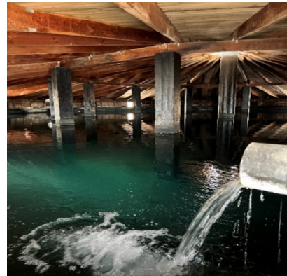
89A Tank NW Tank - Inside
