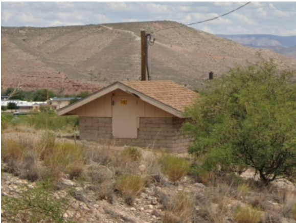
Booster Pump Station Building
