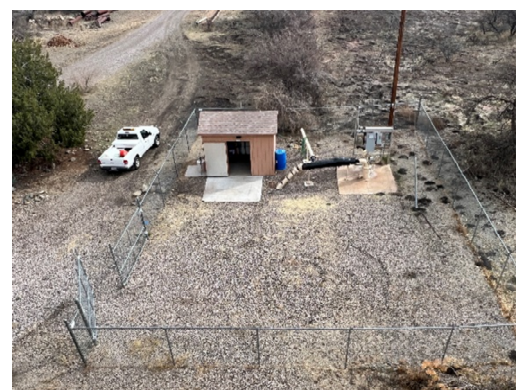
Haskell Springs South Well – Well Site
