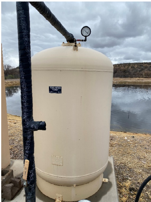
Hydropneumatic Tank
