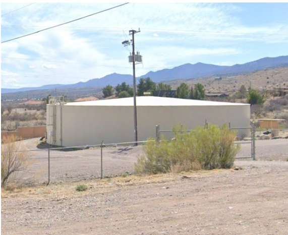
MT Gate Tank – Facing South
