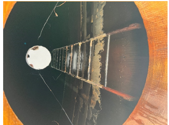
Haskell Springs (South Tank) – Inside Coating
