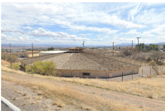
89A Tank NW Tank – Facing South East
