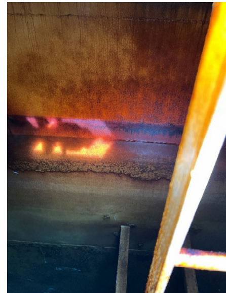
MT Gate Tank – Interior Coating
