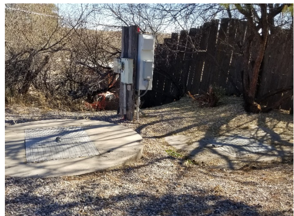
Wet Well and Valve Vault Location
