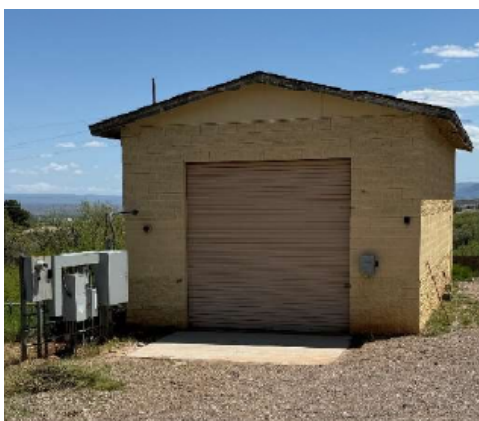
Arsenic Treatment Building
