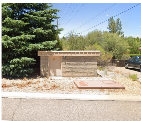
Booster Pump Station Building
