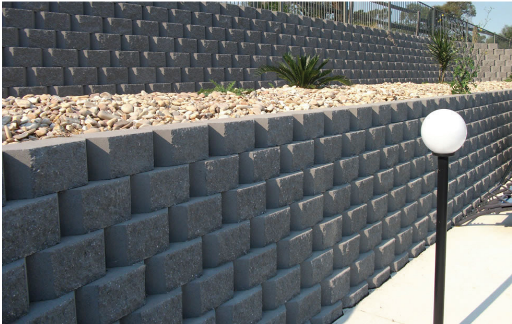
Wall Type 2 - Segmental Block Walls
