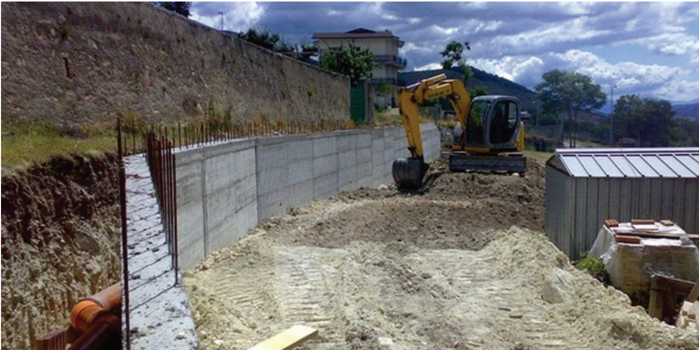
Wall Type 3 - Conventional Cantilever Retaining Wall
