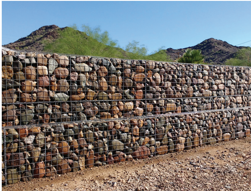
Wall Type 1 - Gabion Baskets
