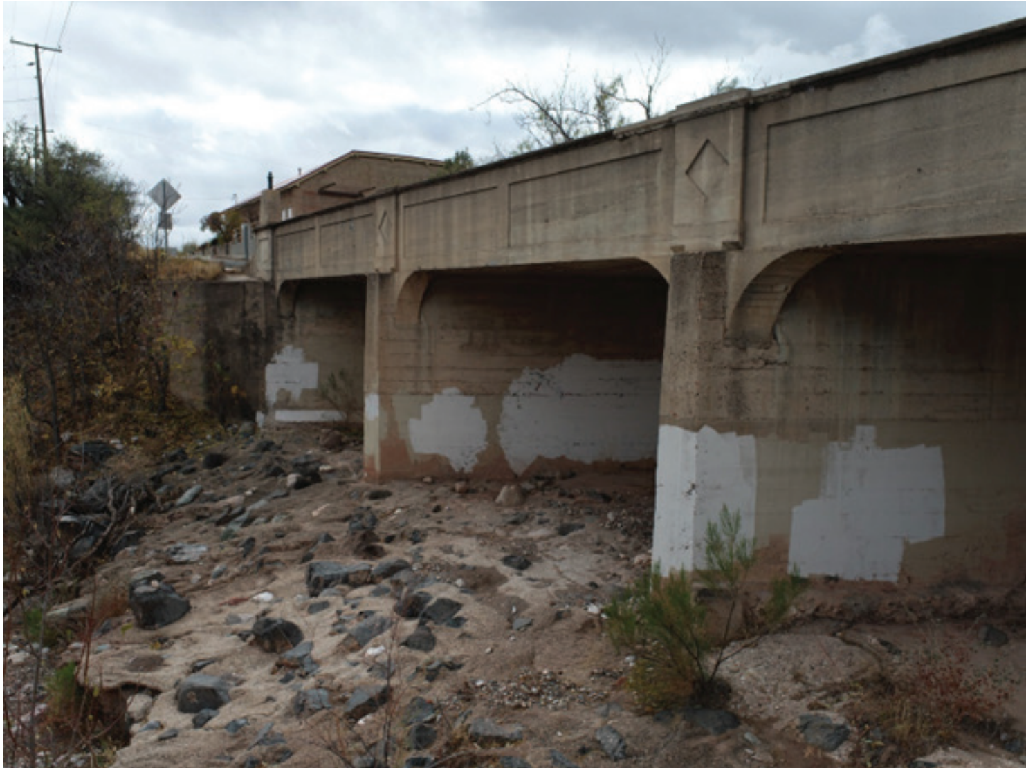
Existing Barrier Rail Rustication
