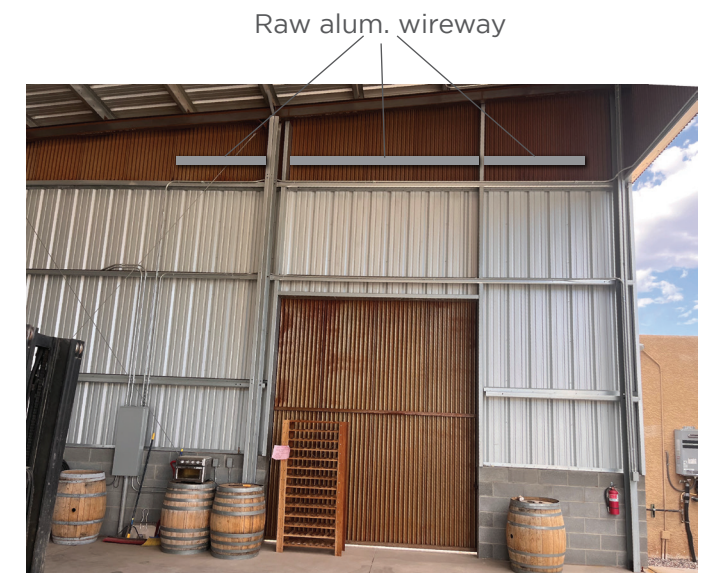
Backside of the wall
