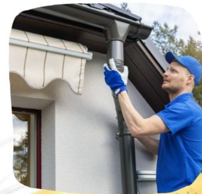
4,000 GAL RAINWATER SYSTEM
